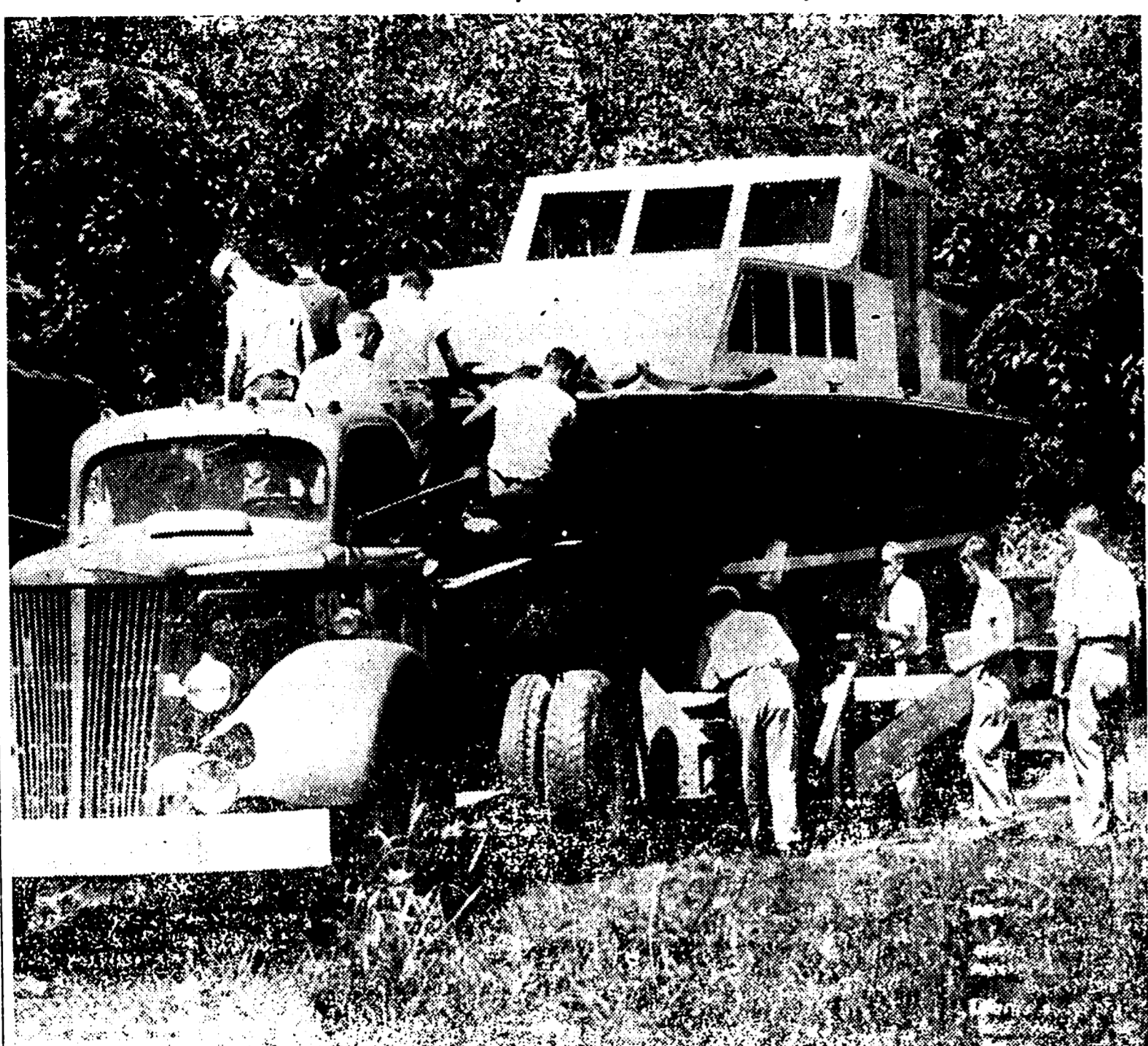
Christened the Leo Maris, a former Navy combat landing craft is loaded on a riggers tractor-trailer to be hauled from Swarthmore to the Sun Shipbuilding & Dry Dock Co. yard, Chester, for launching. Hull was rebuilt and a superstructure added by members of Sea Scout Ship 329, working two years on the project.
