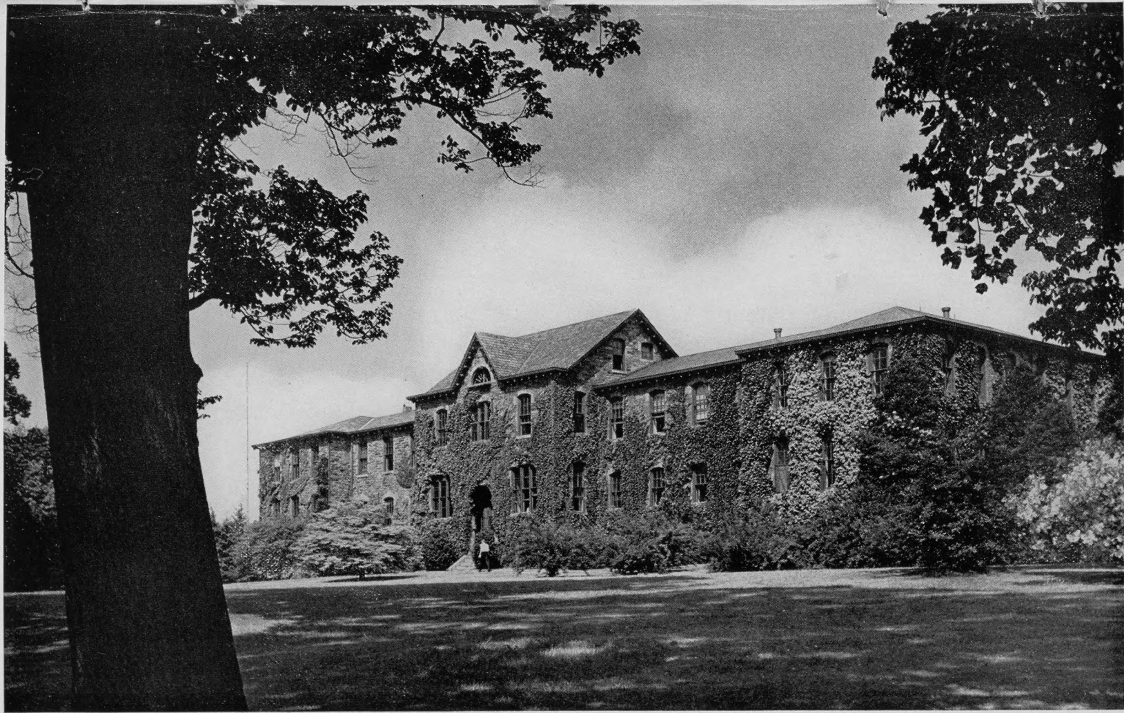
Trotter Hall (a Classroom Building).
