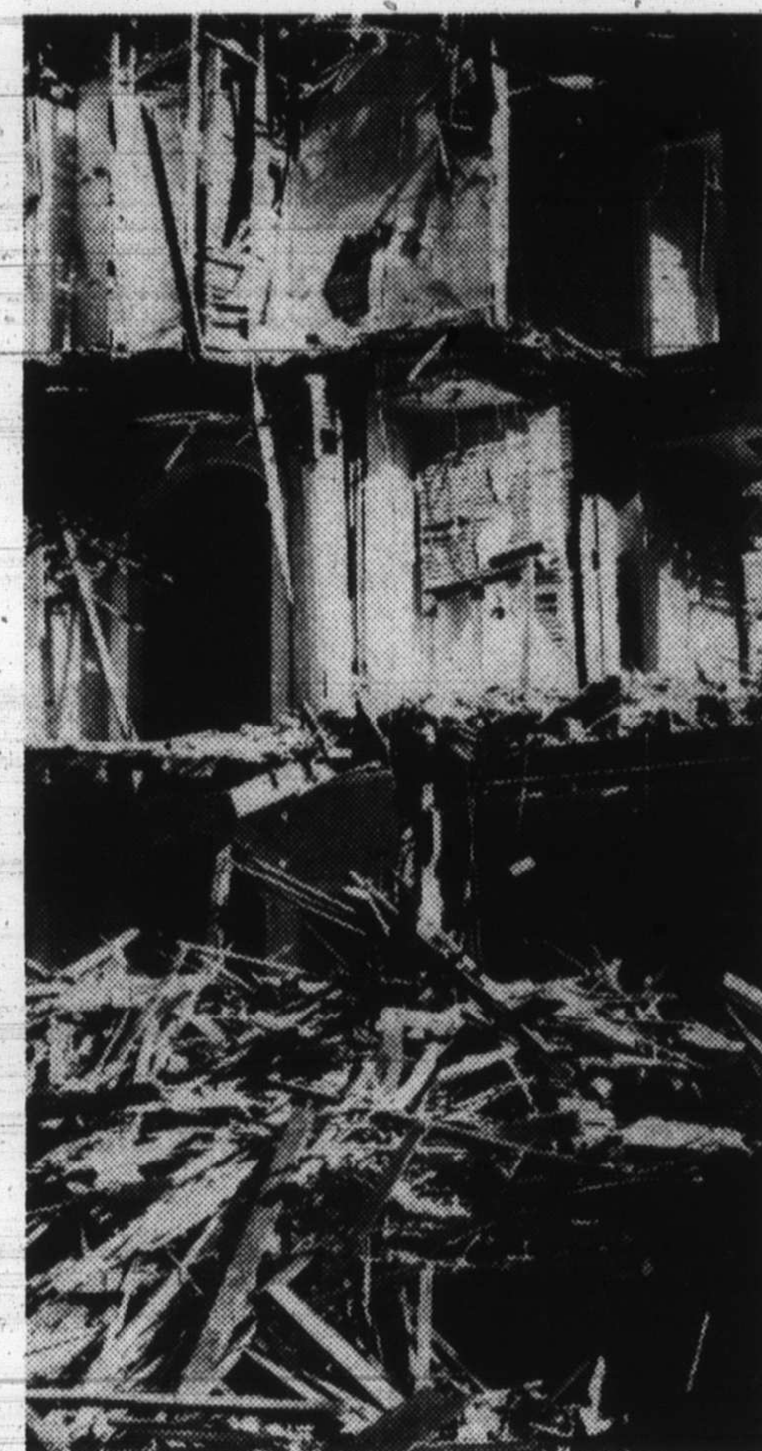
Edifice Wrecked: East House goes down.
